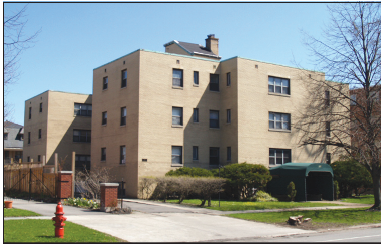
Linwood Manor Apartment Complex, 277 Linwood Ave., Buffalo
